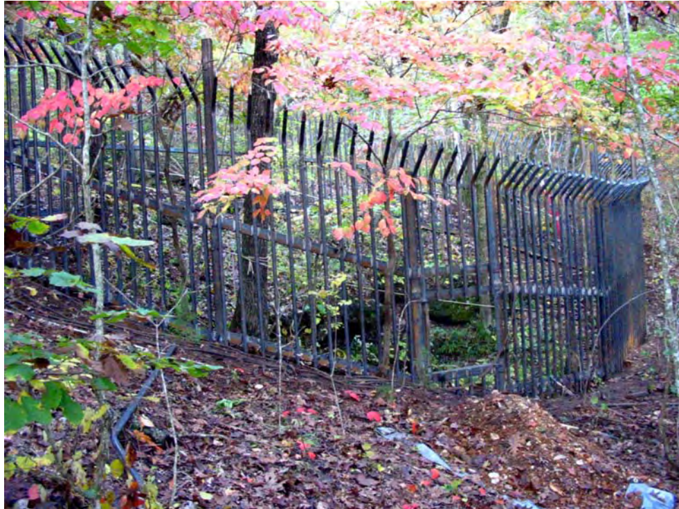
A 10-foot-high, vertical bar fence around a pit entrance in Missouri. The access door is temporarily open. By Jim Kaufmann and Kenny Sherrill.
